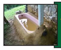
Step 5: do the finish with a mixture of clay and sand (without straw)
