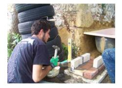
Step 4: build the fire system with bricks and make the extraction system
