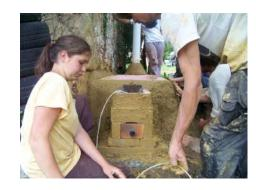
Step 6: wait for the cub to dry (the time to dry depends on the weather) - normally it is around a week
