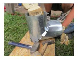
6. Using hammer hit the standing-out parts to connect them with elbow.
