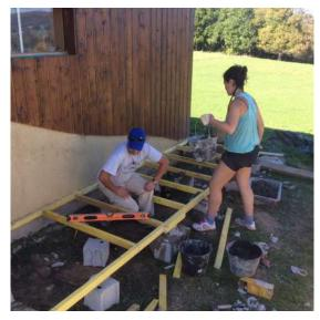
The formwork is ready to welcome the decking woods. Before we screw the planks to the timbers underneath we should have in mind the distance between the planks. In order to achieve this we used little pieces of wood with thickness of 2-3mm, avoiding the expansion of the wood because of the rain and humidity. For an aesthetic result we screw the planks in the same lines.
